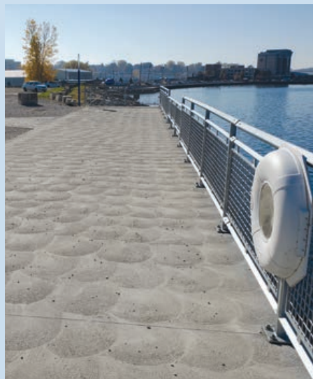
The Holland Street Pier, Erie County, features smooth and open paved surfaces from parking lot to pier and provides lowered railings for anglers to fish from the seated position.
