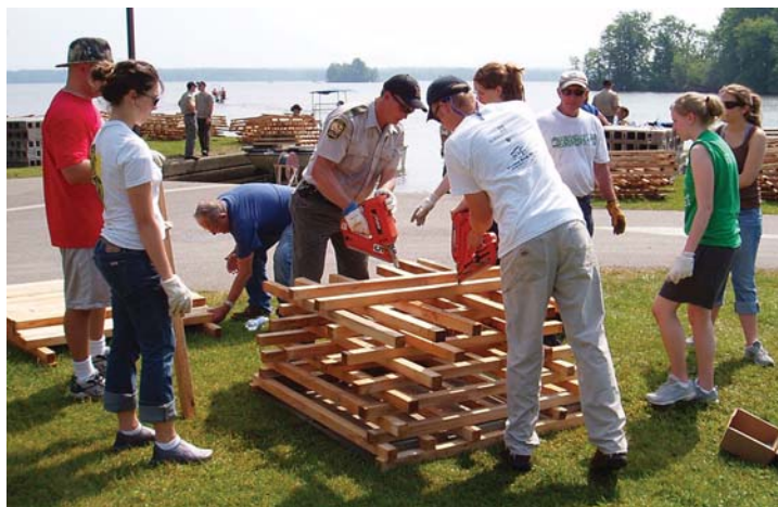
Types of habitat structures might be wooden porcupine cribs that are sunk in a lake to provide fish spawning structure.
