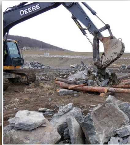
*The Pennsylvania Fish & Boat Commission Division of Construction and Maintenance is often tasked with building large structures called spider humps. Habitat structure construction is executed quickly with heavy equipment like this excavator.*
