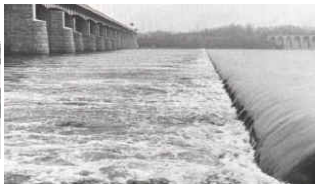
The same low-head dam from an across-the-river view.
