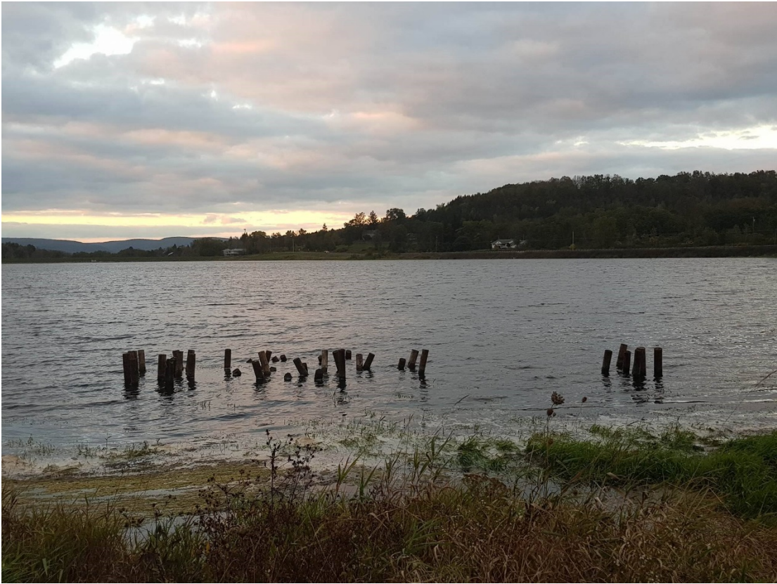
Newly placed post cluster habitat structures at Lake Nessmuk
