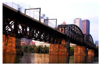
**Figure 7.12.** Featuring bridge piers constructed of hand-cut sandstone, the Panhandle Bridge across the Monongahela River affirms Pittsburgh's moniker the "City of Bridges" (from Pittsburgh Bridges 2010).
