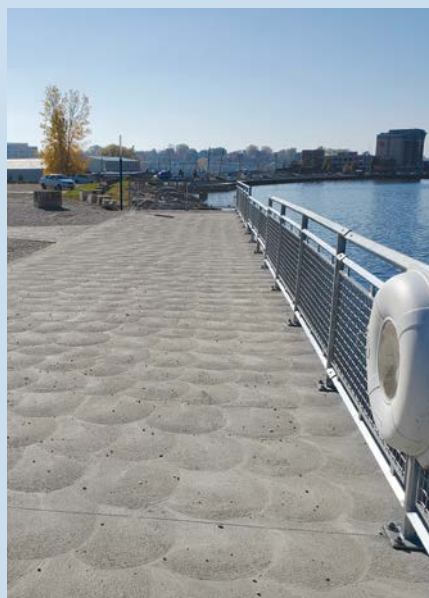
The Holland Street Pier, Erie County, features smooth and open paved surfaces from parking lot to pier and provides lowered railings for anglers to fish from the seated position.
