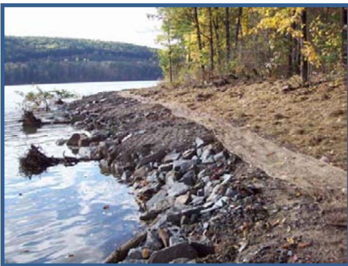
Both Cowanesque (left) and Hammond (right) Lakes in Tioga County had some shoreline erosion issues that were treated with these root wad and stone-framed deflectors. Each lake also received Short Vertical Plank structures as off-shore habitat as part of the cooperative habitat project between the US Army Corps of Engineers, Tioga County Bass Anglers and PFBC.
