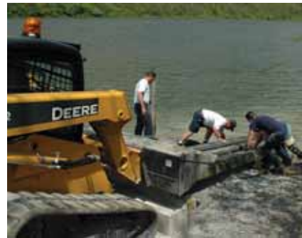
Boat slide installed at Lake Gordon, Bedford County.
