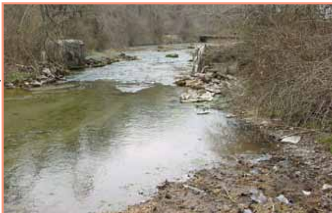
Remains of the Piper Mill Dam with a portion of the former impoundment in the foreground as it appeared in 2007.
