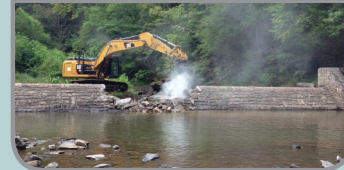
Restoring habitat connectivity
