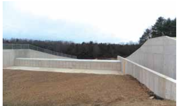
Colyer Lake Dam, Centre County
