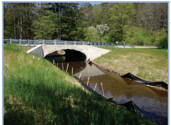
Trout Unlimited removed a fish passage barrier through replacement of an undersized, metal pipe culvert with a bottomless arch at bankfull width on Little Lyman Run, a wild Brook Trout tributary to Cross Fork Creek, Potter County.
