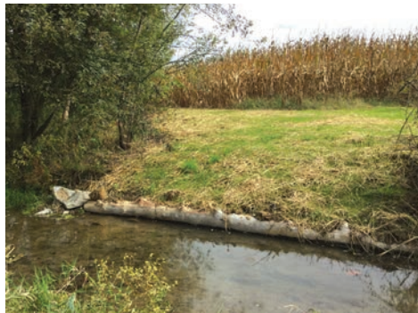
Habitat structures slow bank erosion, which reduces the amount of sediment and nutrients entering the stream and, ultimately, the Susquehanna River.
