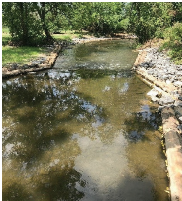
Buffalo Creek, Union County
