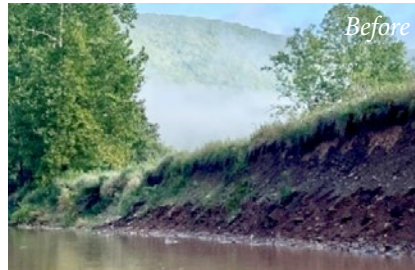
A 16-foot-high, eroded streambank on Little Pine Creek, Lycoming County.
