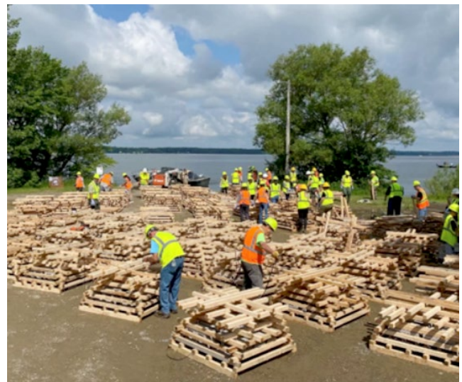
Volunteers construct 130 wooden fish habitat structures for Pymatuning Reservoir, Crawford County.
