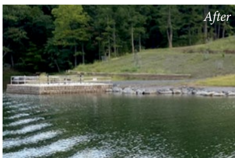
A stabilized shoreline with stone deflectors, new fishing pier, and ADA accessible walking path at Raystown Lake.
