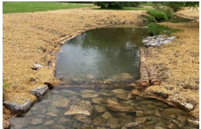
A log-frame cross vane structure on Buffalo Creek, Butler County.
