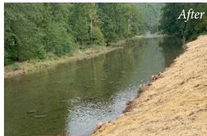
The restored, stabilized streambank on Little Pine Creek.
