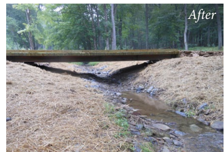
West Branch Hicks Run with new timber deck bridge installed.
