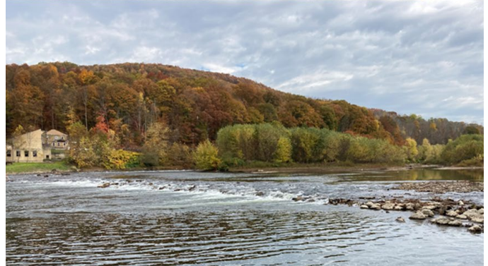
The removal of Oakland Dam on the North Branch Susquehanna River, Susquehanna County.
