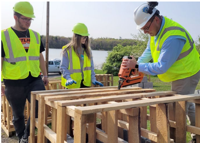
Students constructing habitat structures at Somerset Lake, Somerset County.
