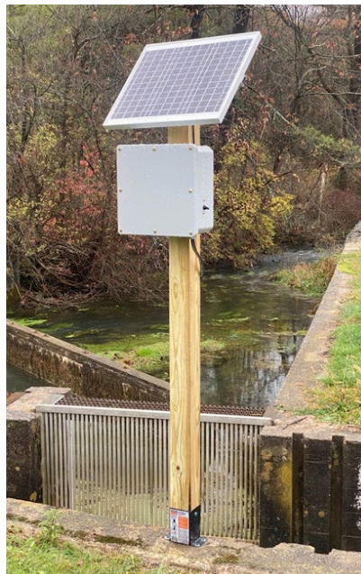
New Zealand Mudsnaill solar powered, electric barriers were installed in channels at the Benner Spring State Fish Hatchery and Pleasant Gap State Fish Hatchery.
