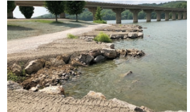
Streambank stabilization at Lake Arthur, Moraine State Park, Butler County.
