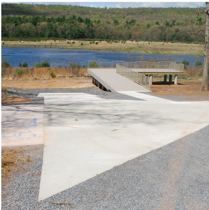
The Americans with Disabilities Act (ADA) accessible pier at Meadow Grounds Lake, Fulton County.
