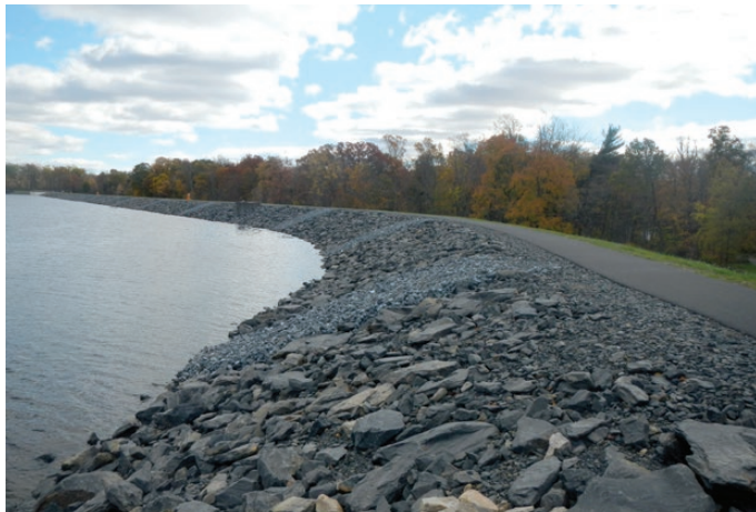
Minsi Lake Dam, Northampton County
