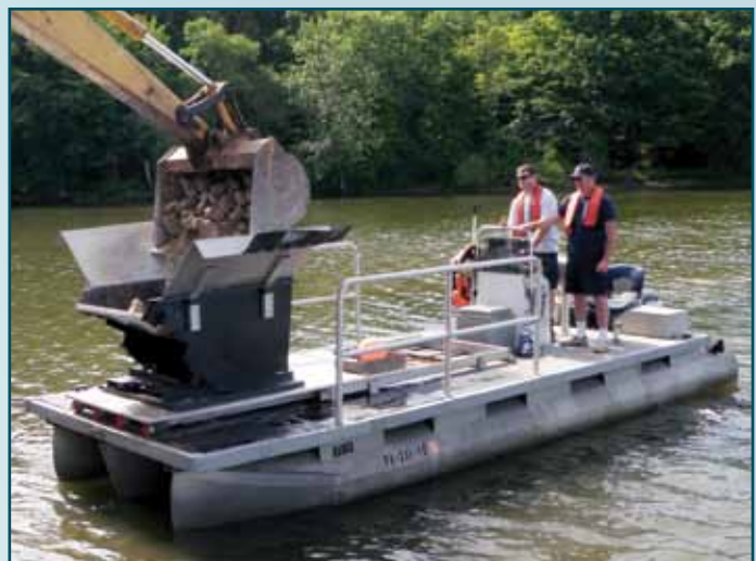
Rocks and gravel are loaded and then discharged from dump boats.
