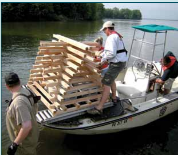
The rollers on crib boats make it easier to install porcupine cribs.
